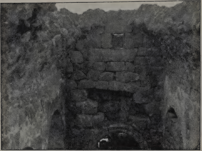
FIG. 105.—No. 16, W. end of nave, showing door into narthex.
